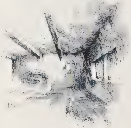
No. 7.—A Bedroom, Livesey Hall.
